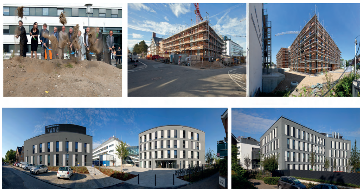
Figure 3. Snapshots from the construction period at MPI CEC 2017-2022.
